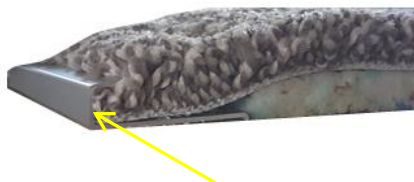
Tile edging trim –Trim the carpet into end.
