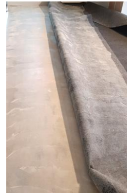
Illustration 3: Adhesive transferred to the carpet backing
