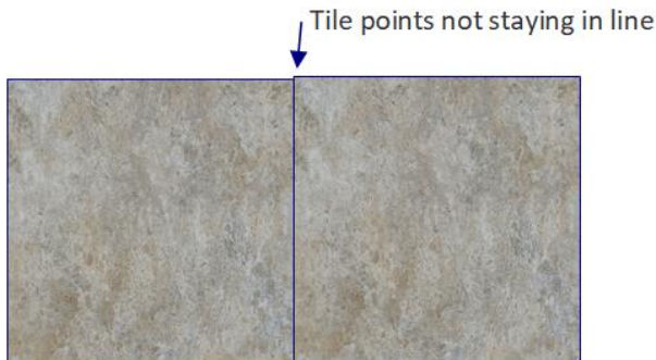
Illustration 1: Tile points not lining up
