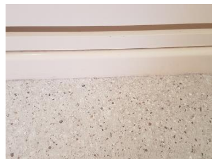
Photo 4 - After vinyl is fitted any excess silicone that squeezes up is removed.
