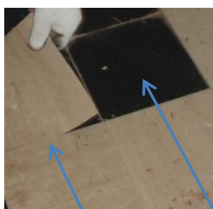
Photo 3 Vinyl asbestos tiles
