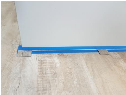
Photo 1 - Setting the bead width.
