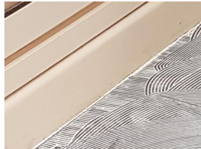
Photo 3 Silicone to the shower/floor junction.
