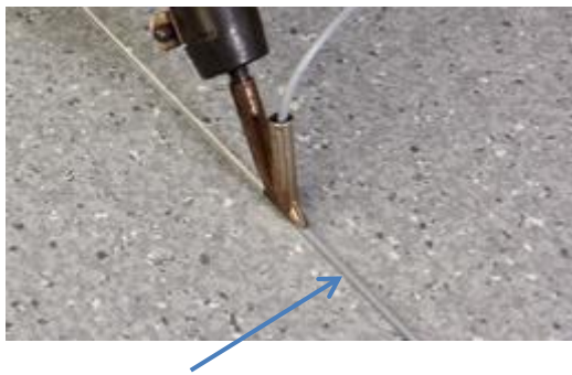
A slight wash of melted weld rod rising at the edge of the weld
