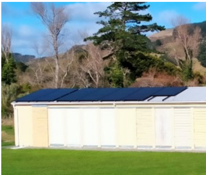
The test building housing the hot water systems under investigation on a sunny winter's day. Three of the hot water systems are connected to the solar photovoltaic panels on the roof
