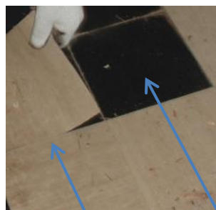
Photo 3 Vinyl asbestos tiles
