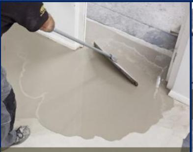
An epoxy moisture barrier will need a cementitious levelling compound to allow the water in the adhesive to soak into the compound: Ardex
