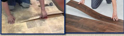
Due to the make up of vinyl (PVC, plasticiser) the common adhesive used is Acrylic based. Acrylic is part of the plastic family so it matches the make up of vinyl.
