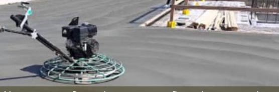
New concrete floors that are power floated to a smooth shiny finish will need grinding to open up the pores
