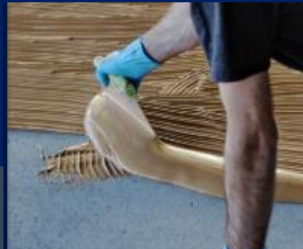
Moisture Cure Polyurethane adhesive - flexible for installing Timber flooring
