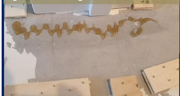
Fast setting- used to fix carpet gripper
