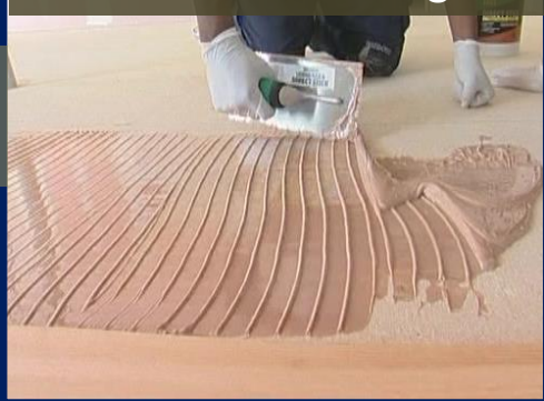
Moisture Cure Polyurethane adhesive - semi rigid foaming
