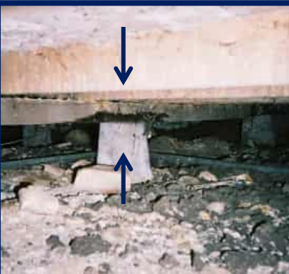
Rotten joists /bearers
