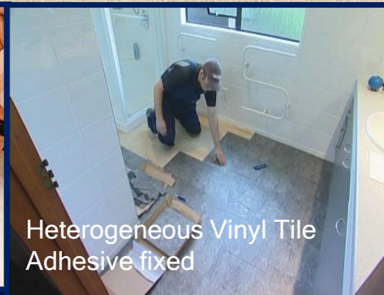
Using a trimming tool or a knife to cut in
