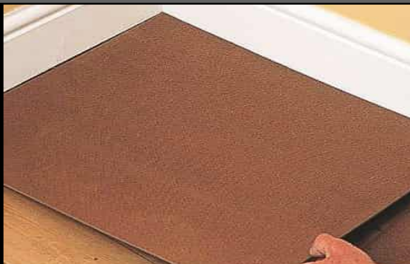
Thin Board - fitted as an underlayment as preparation for vinyl floor coverings
