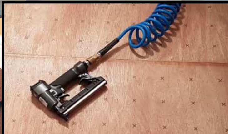
Thin Board - fitted as an underlayment as preparation for vinyl floor coverings
