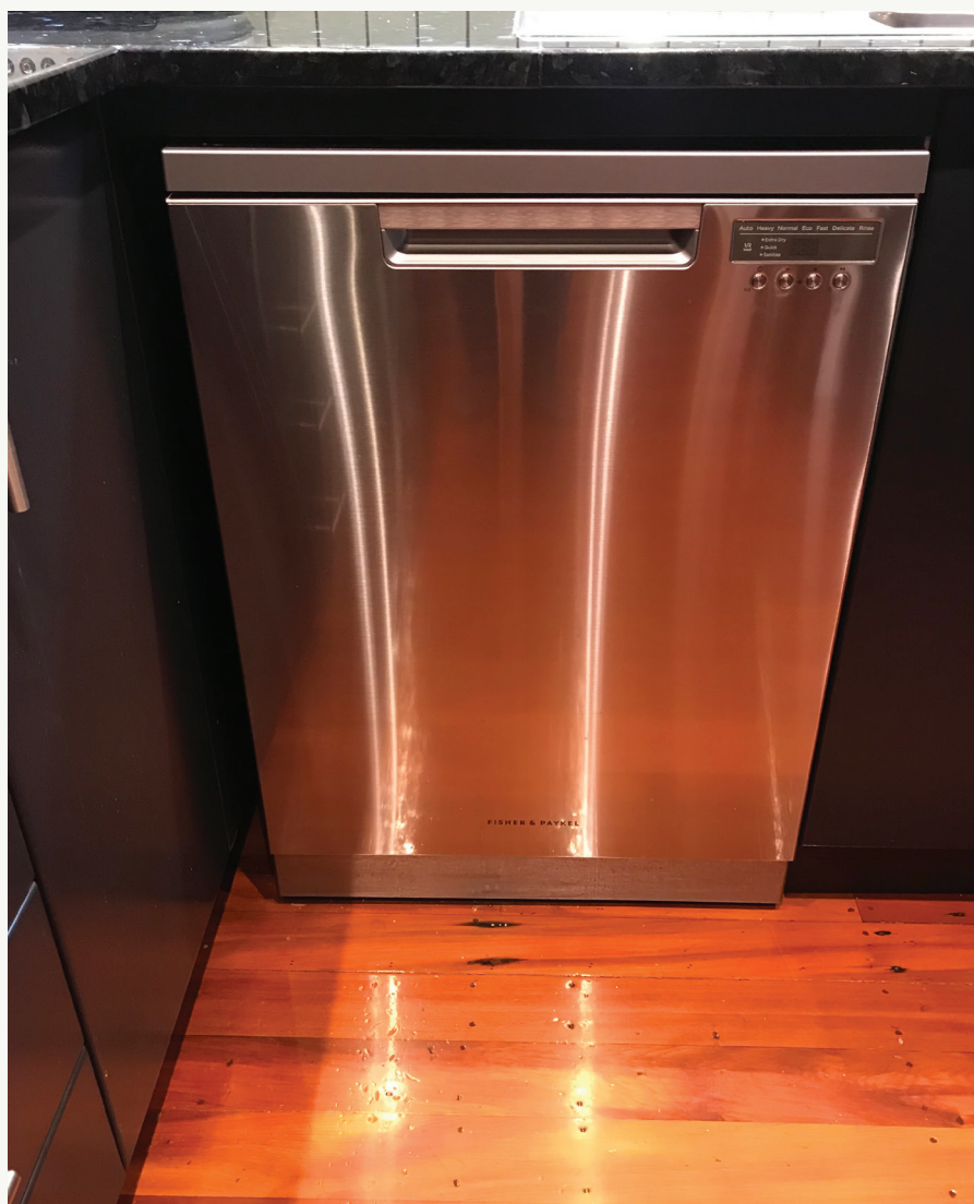
Figure 1: Mātāi timber flooring that has stood up well to splashes and occasional floods over 25 years.
